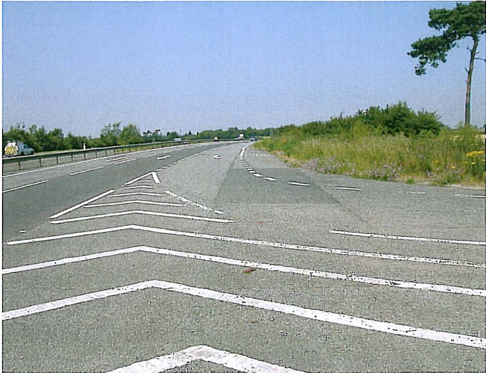
Photograph 2: View of A14 deceleration lane to Croft Lane.
