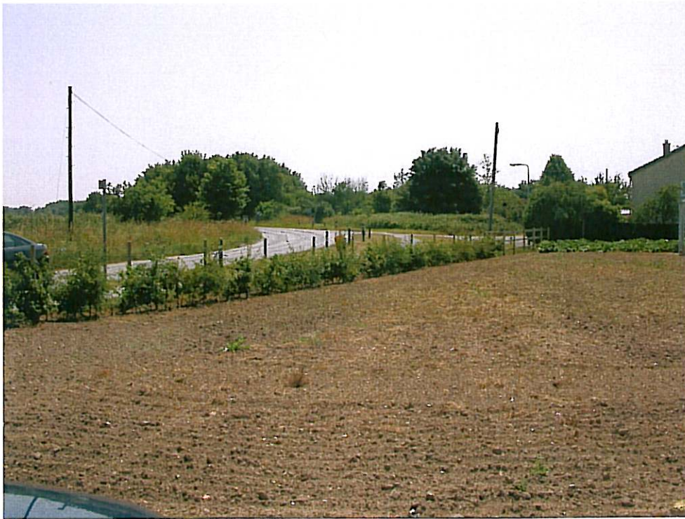
Photograph 5: Corner where access to footbridge meets Kirton Road.
