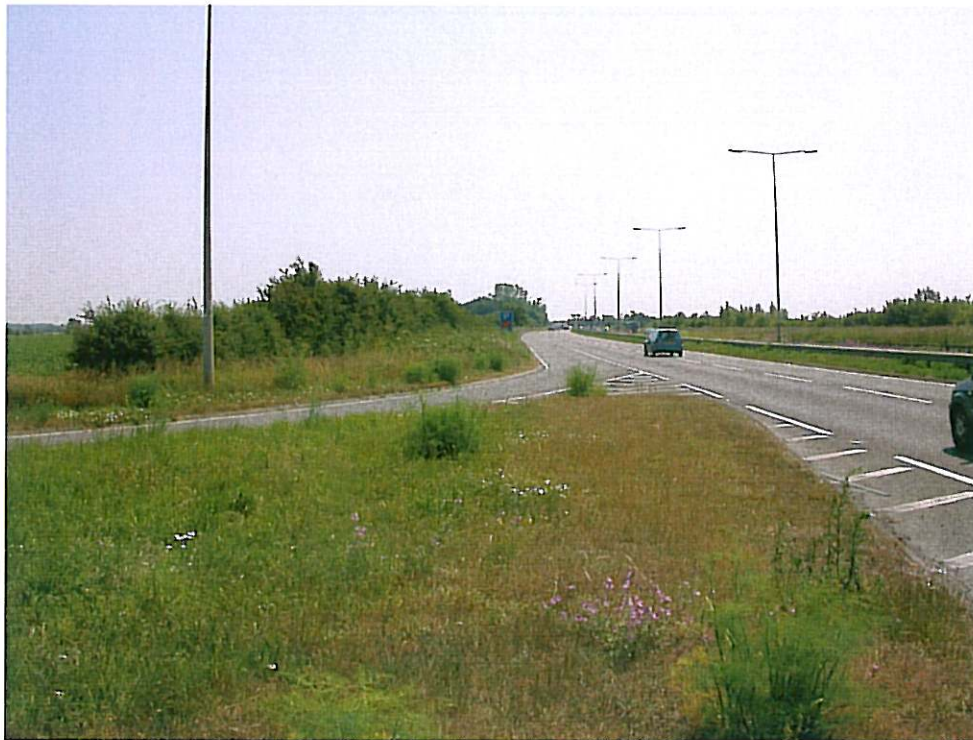
Photograph 3: View A14 acceleration lane from Croft Lane.
